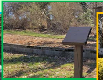
Cinder block retaining wall
