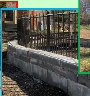
Block wall to level picnic area
