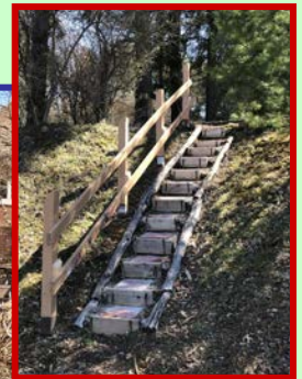
Steps & handrail to upper lawn
